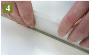
Roll board to fold tape over bevelled edge
