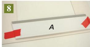
Cut first piece, A, longer than longest opening. Temporarily position with tape
